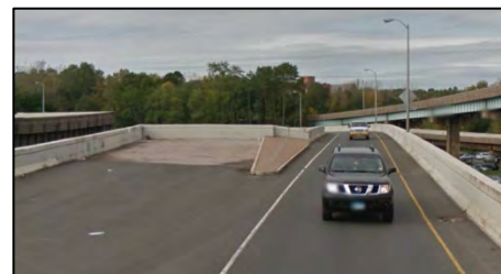
Interchange 46 – Eastbound On-Ramp 'Stub'
