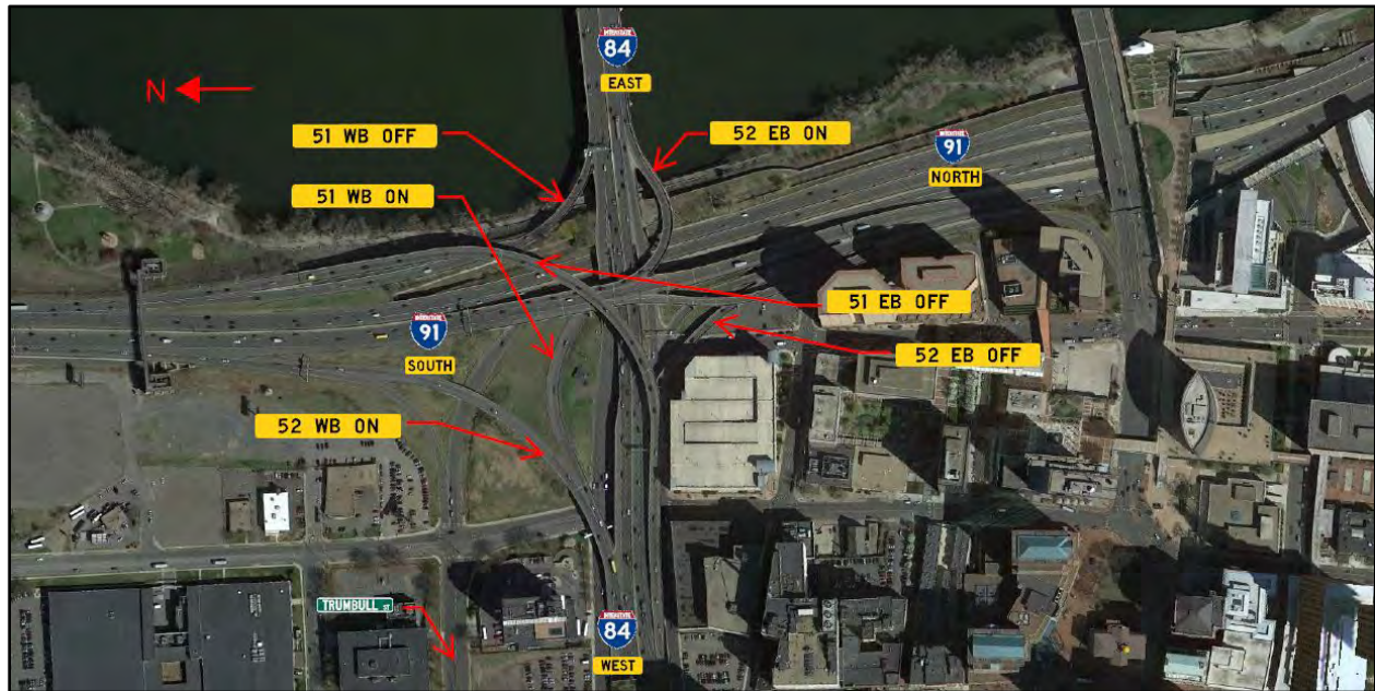
Figure 2-54: Interchanges 51 and 52 (Interstate 91)
