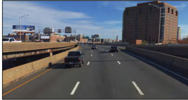
Longitudinal Concrete Barrier along Both Sides of Mainline
